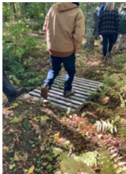
Bridges can be an expensive trail enhancement, unless you have access to a shipping pallet
